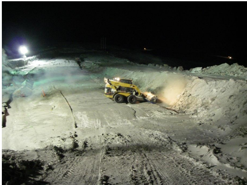
Photo 8: Additional cleaning of the frozen core material at night.
