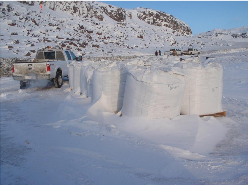
Photo 4: Bentonite chips staged near the diversion berm in preparation for liner key-in.
