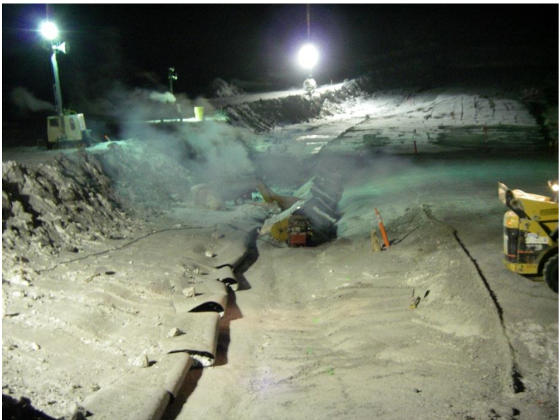
Photo 10: Hoarding tents thawing material above the GCL.
