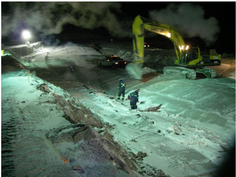
Photo 9: Labourers cleaning next to the GCL. The excavator peeled back loose FCM.
