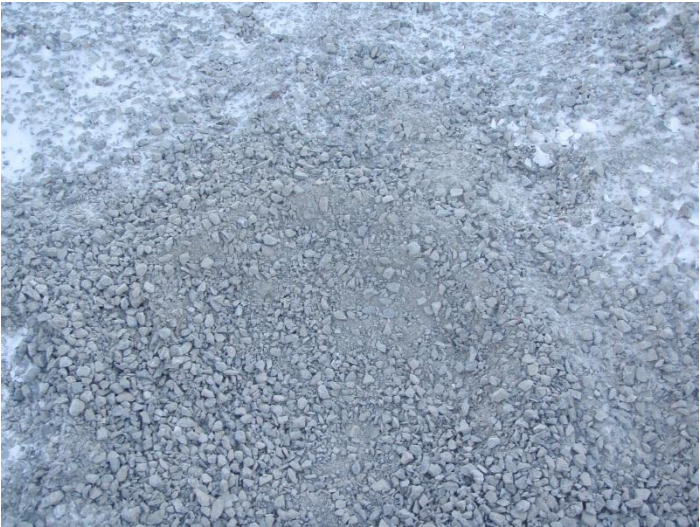
Photo 5: Close-up of the Doris North Diversion Berm key-trench. Floor has been kicked loose to illustrate presence of fines.
