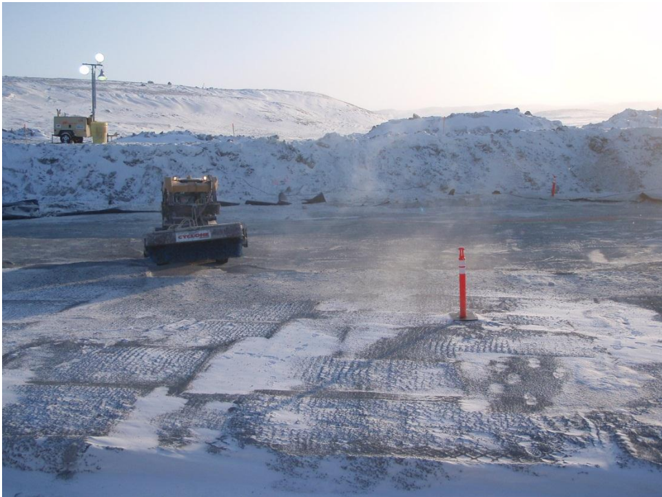
Photo 6: Skidsteer equipped with broom attachment cleaning loose gravel from frozen core area.
