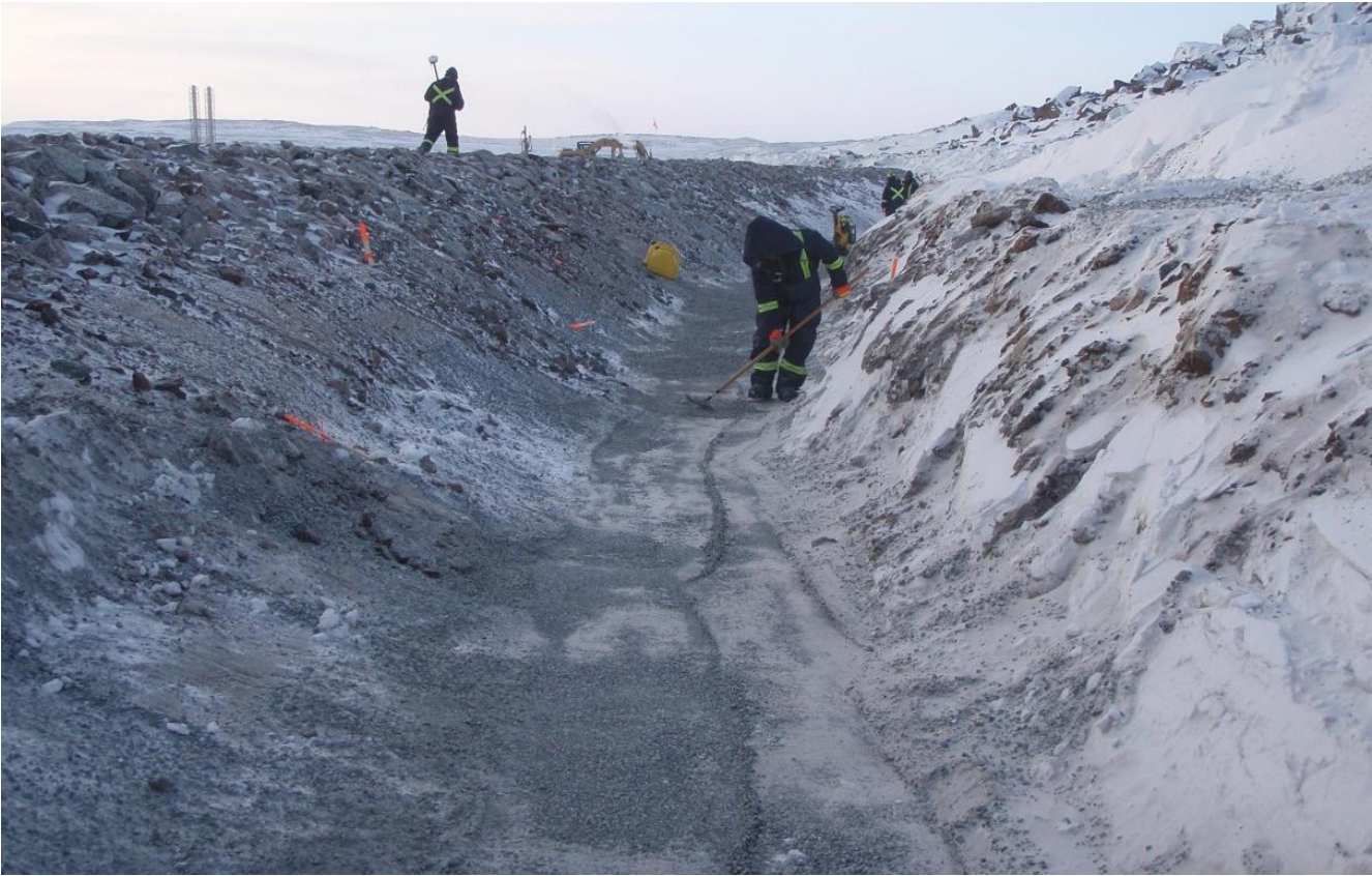
Photo 3: East end of the Doris North Diversion Berm looking east. Labourers raking and compacting the key-trench with a plate tamper.
