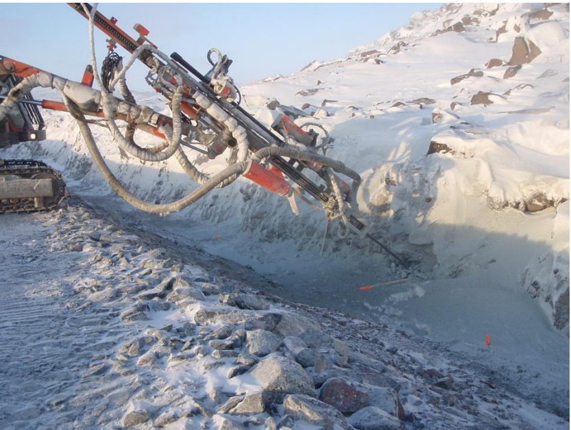
Photo 2: Drill honey combing bedrock for removal at the Doris North Diversion Berm.
