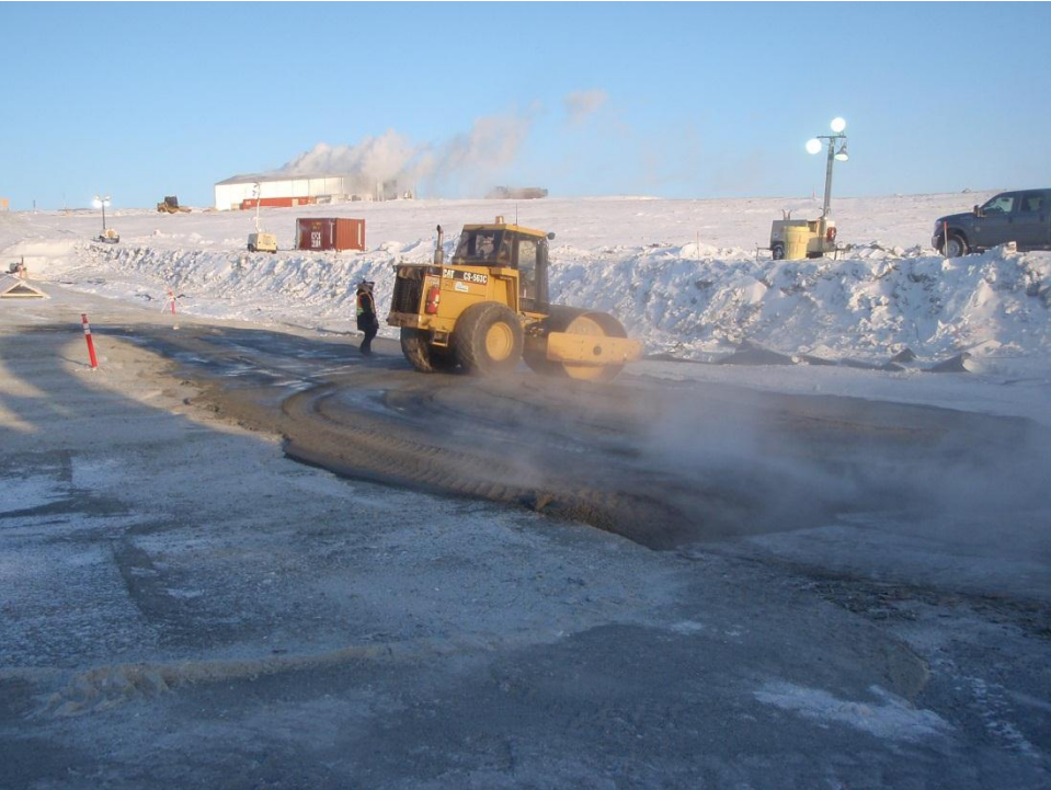
Photo 7: Vibratory compactor packing today's lift of FCM. Note the operator's close attention to not drive on the unfrozen material in the foreground.
